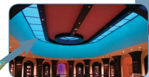
Atlantis III Resort and Spa The Bahamas Design: Lighting Design Alliance A project-specific housing positions two Pixels about 18 inches (457 mm) apart. The housings are installed in the horseshoe-shaped ceiling, ensuring a smooth backlighting effect across the acrylic lenses.
