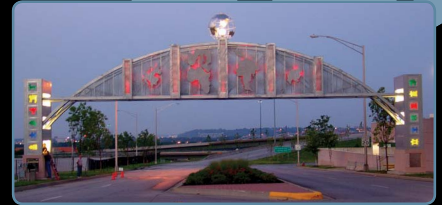
Minnesota Avenue Bridge Kansas City, Kansas
